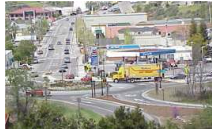
Idaho-Maryland/East Main St. Roundabout at SR 20/49 Freeway
