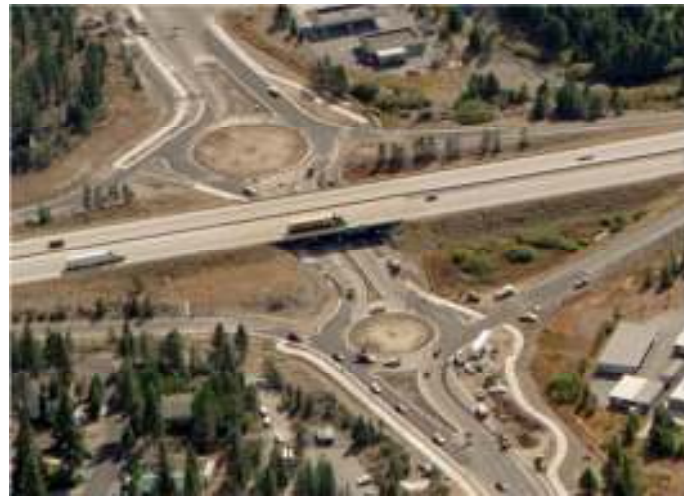
Truckee Dual Roundabouts at the I-80/SR 89 Interchange
